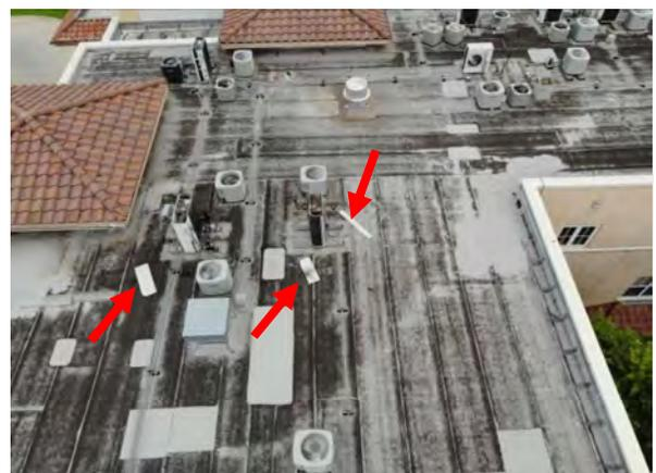
**Photo #36** View of metal debris scattered on the roof.
