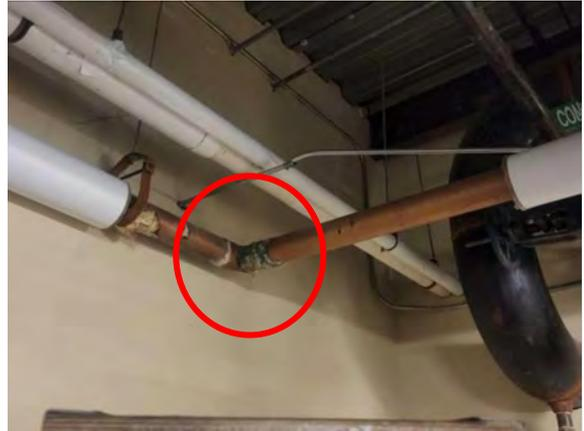
**Photo #98** Electrolysis corrosion on copper water distribution piping.
