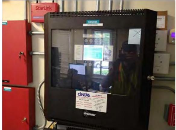
**Photo #142** Fire alarm control panel.
