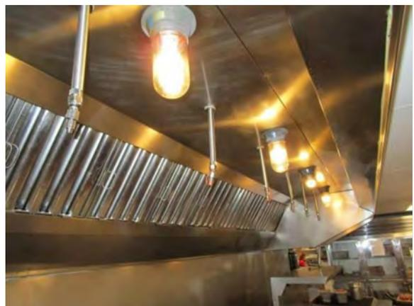
**Photo #156** Cooking area exhaust hood with fire suppression system nozzles.
