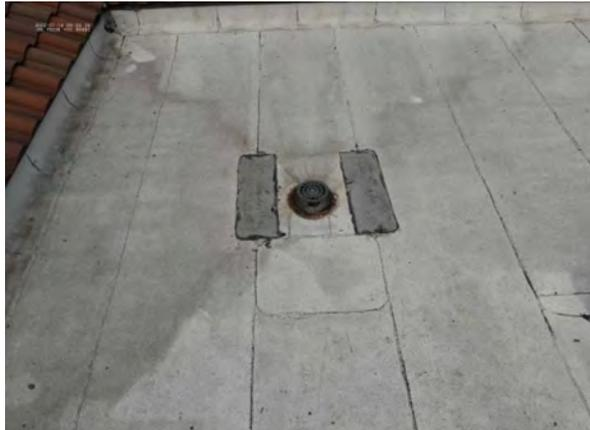
**Photo #43** Low slope modified bitument roof drain.
