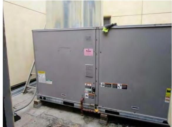
**Photo #116** Packaged DX roof-mounted unit (RTU) for Greenhouse.
