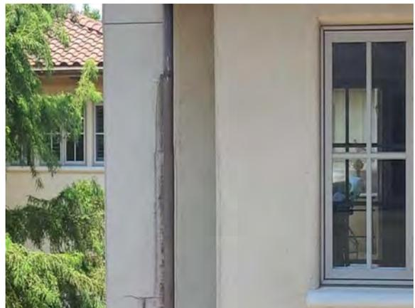
**Photo #54** View of damaged stucco façade caused by broken downspout.
