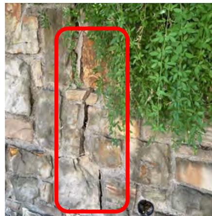
**Photo #66** Mortar joint crack in retaining wall
