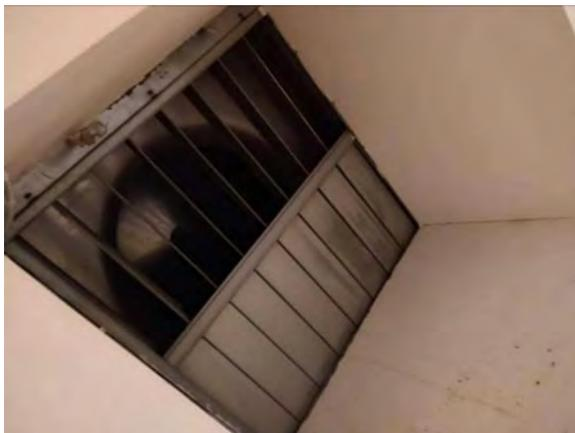
**Photo #161** Smoke damper stuck open in parking structure.
