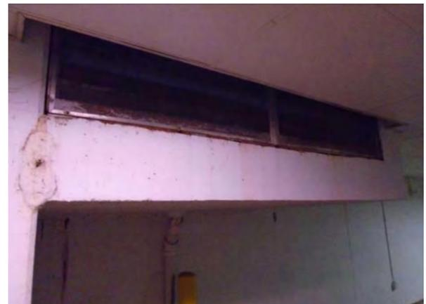
**Photo #162** Outside air intake for parking structure ventilation.
