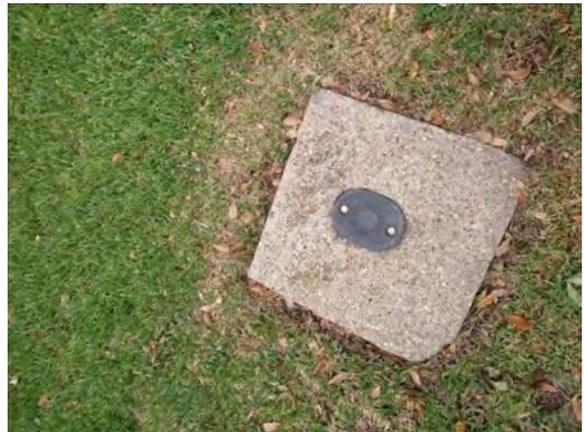
**Photo #154** Typical sanitary sewer clean out for building.
