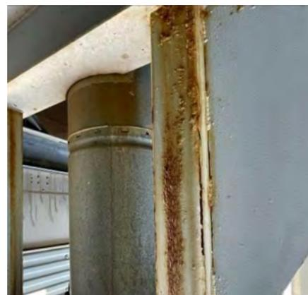
**Photo #60** Cooling tower structure shows deterioration.
