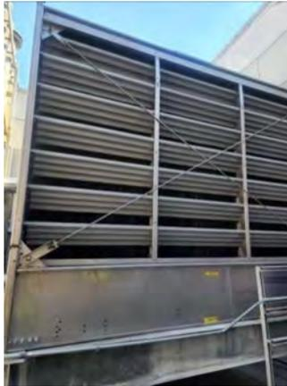
**Photo #93** Cooling Tower for water source heat pump system.
