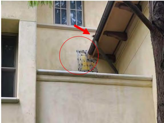
**Photo #49** View of debris clogging downspout and wall repair. Note wall repair and repainting.
