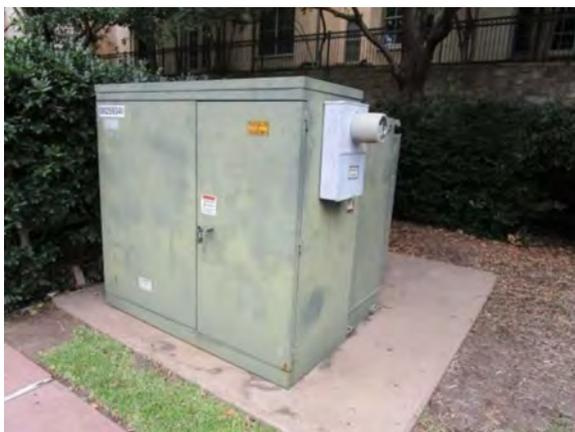
**Photo #149** Typical utility transformer and electric meter for electrical service to the building.
