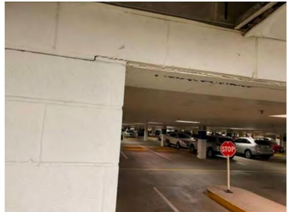
**Photo #58** Joint of Phase II with Phase I in main parking structure showing crack on CMU wall and water damaged. beam.
