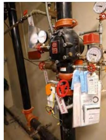
**Photo #138** Dry-type fire suppression riser for parking garage.
