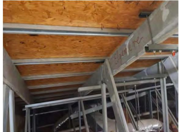
**Photo #22** View of OSB roof deck supported by metal framing.
