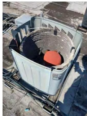
**Photo #114** Older condensing unit with missing condenser fan and motor.
