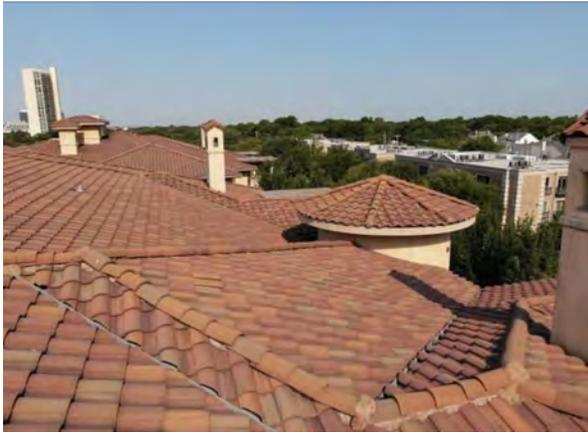
**Photo #21** Close view of concrete tile roof.
