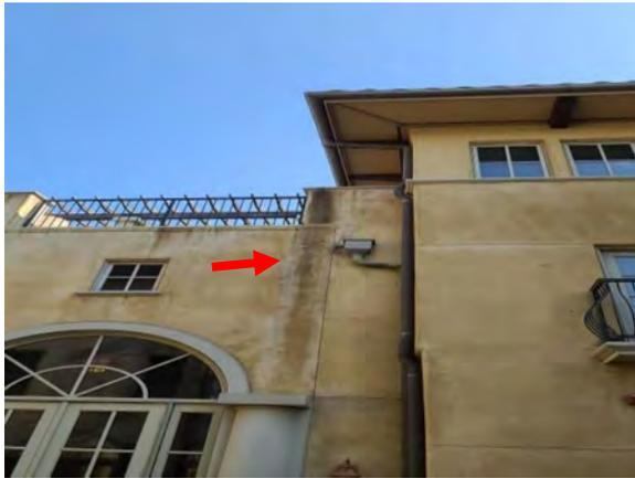
**Photo #51** View of staining on stucco façade.
