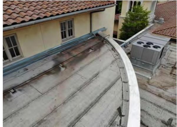
**Photo #38** View of staining on the modified bitumen roof.
