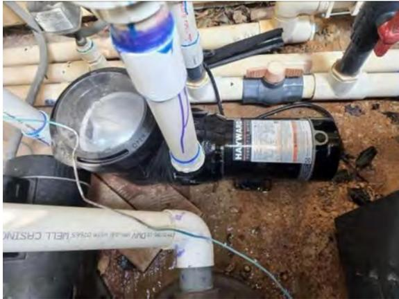
**Photo #109** Leaking pool circulation pump.
