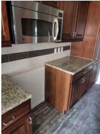
**Photo #129** Typical dwelling kitchen exhaust system with built-in to over range microwave.
