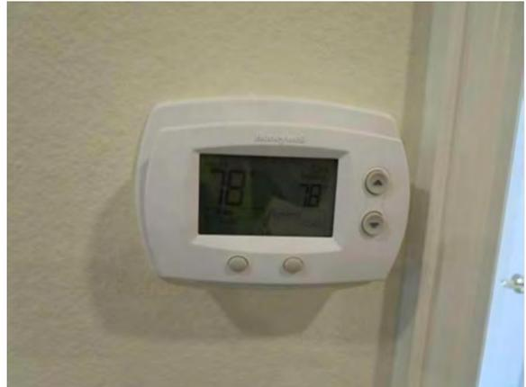
**Photo #122** Stand-alone thermostat for WSHP and DX split systems in dwelling units.
