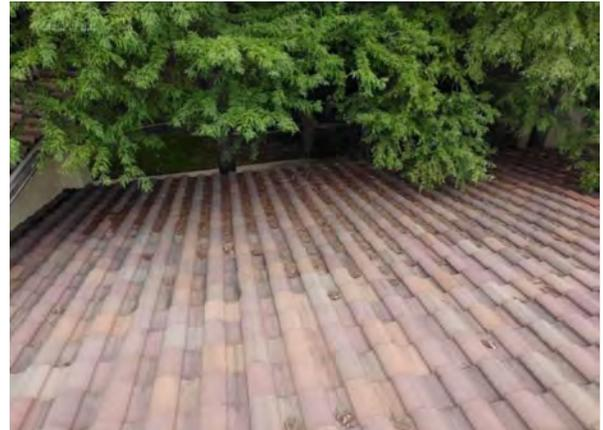
**Photo #26** View of debris build up on roof. Note tree encroachment of roof.
