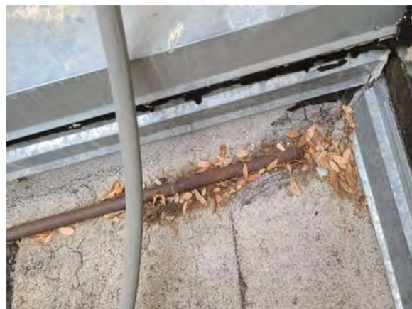
**Photo #41** View of cracking in modified bitumen membrane.
