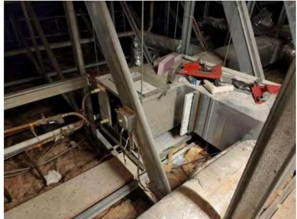
**Photo #112** Ceiling hung water source heat pumps (WSHPs) for dining and other common areas.
