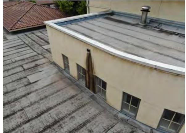
**Photo #46** View of water staining to wall surface from scupper.
