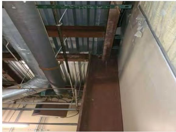
**Photo #33** View of metal low slope roof deck.
