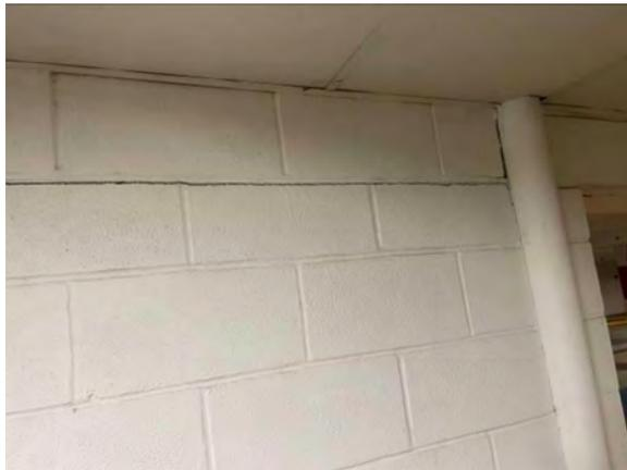
**Photo #57** Joint of Phase II with Phase I in main parking structure showing crack on concrete masonry unit (CMU) wall.
