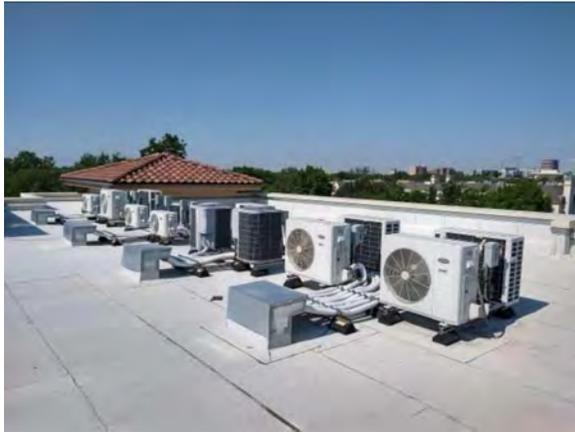
**Photo #115** Newer DX split system condensing units.
