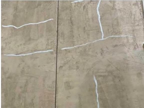
**Photo #67** Repaired cracks in stucco at several locations.
