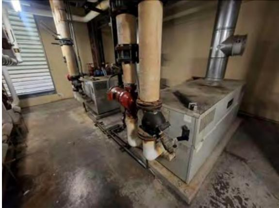
**Photo #97** Auxiliary heating hot water boilers for water source heat pump system.
