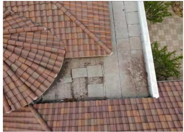
**Photo #34** View of multiple roof patches on the modified bitumen roof.
