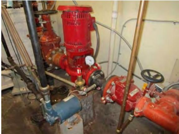
**Photo #139** Fire sprinkler suppression pump.
