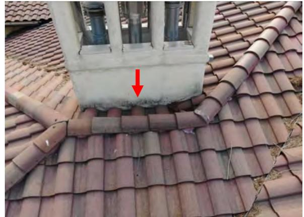
**Photo #44** View of water staining at the base of the chimney.
