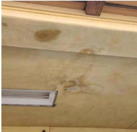
**Photo #55** View of staining on ceiling.
