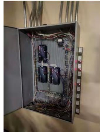
**Photo #146** Reliable Controls field controllers for central plant.
