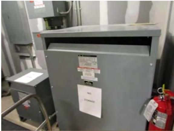
**Photo #145** Typical step-down transformer for lighting and plug loads.
