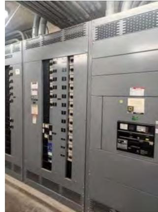
**Photo #106** One of eight main electrical service gear panel boards.
