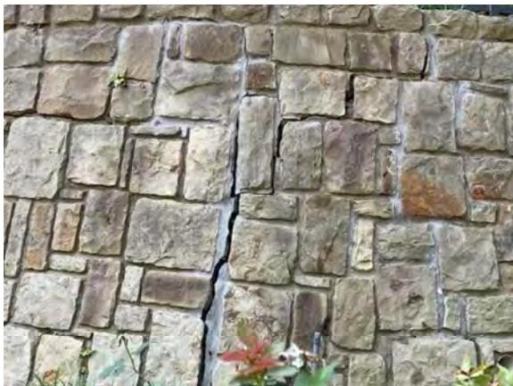
**Photo #65** Mortar joint crack in retaining wall.
