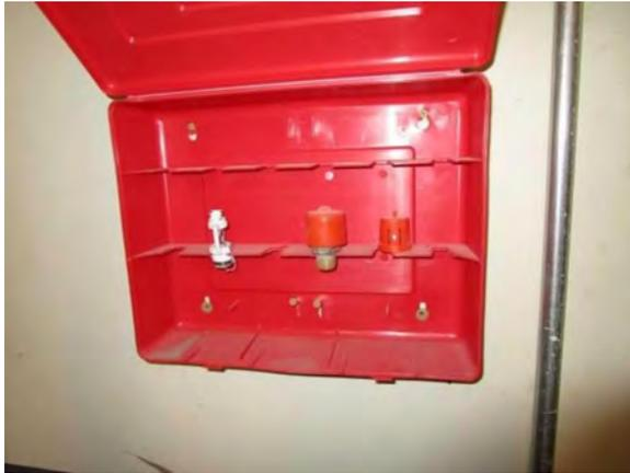
**Photo #141** Spare fire sprinkler head storage case.
