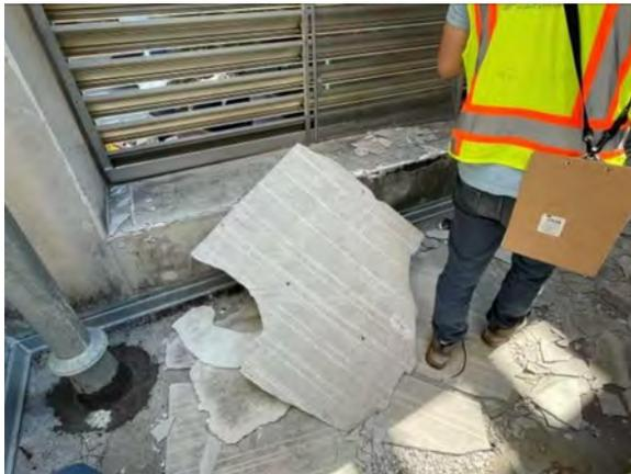
**Photo #63** Broken wall panels on floor in the cooling tower.
