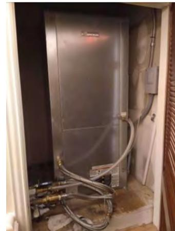
**Photo #118** Newer WSHP (vertical orientation) in mechanical closet for dwelling unit.
