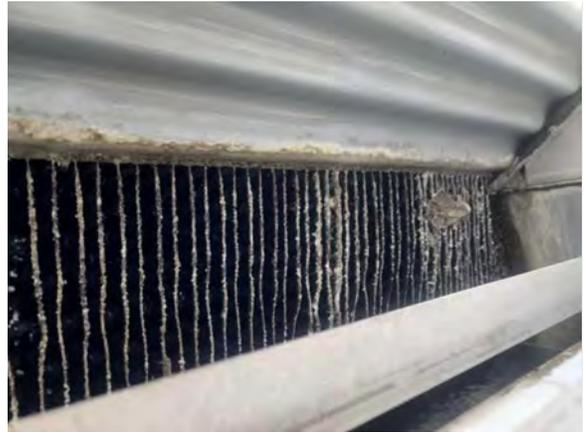
**Photo #94** Excessive scale built-up on cooling tower fill and louvers. Note: "Cooling Tower Fill" is media (plastic typically) used to exchange heat between the entering and leaving cooling tower water with the air being blown across it
