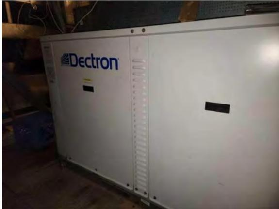
**Photo #111** Dectron dehumidification system for pool area.
