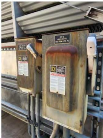
**Photo #95** Original to construction electrical disconnect for cooling tower fan.
