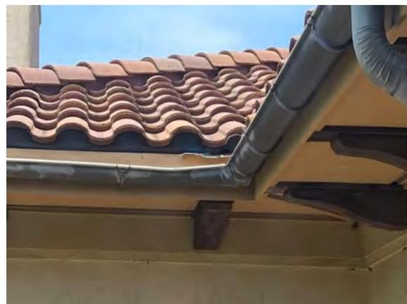
**Photo #47** View of staining on gutters from overflowing water.
