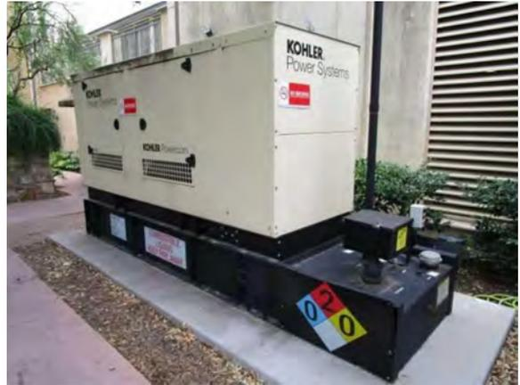
**Photo #152** Emergency generator for fire and life safety systems.
