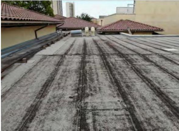
**Photo #31** Close view of modified bitumen roof.
