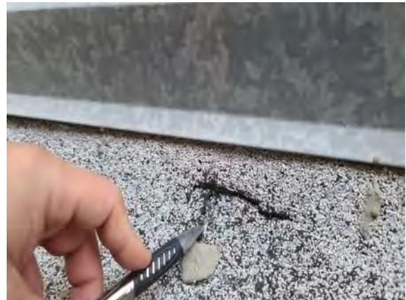
**Photo #40** View of hole in modified bitumen roof membrane base flashing.
