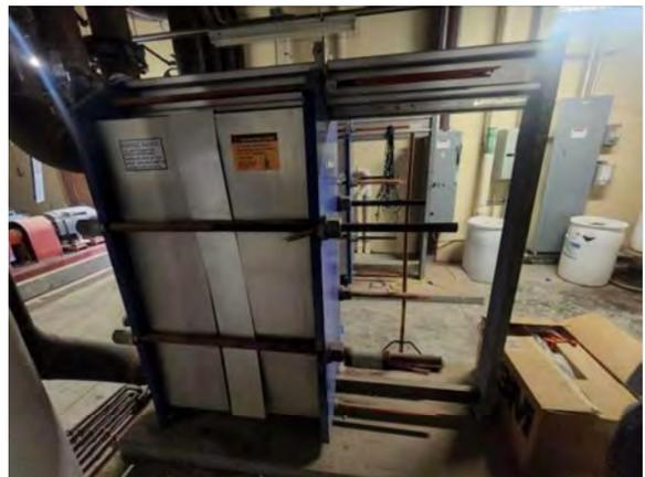
**Photo #102** Plate-frame heat exchanger.
