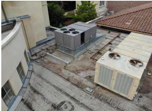
**Photo #39** View of staining from standing water on the modified bitumen roof.
