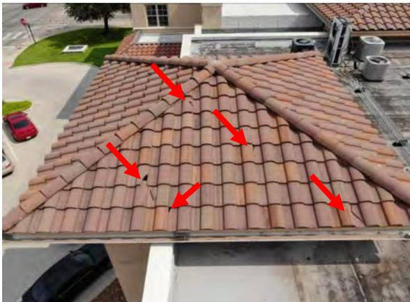
**Photo #23** View of broken tiles on roof. Located periodically through site.
