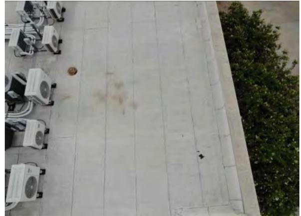
**Photo #32** Close view of modified bitumen roof.
