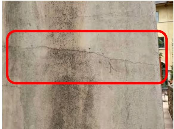
**Photo #70** Random cracks in stucco in general.
