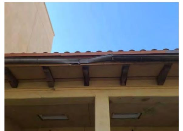
**Photo #48** View of severely damaged gutter.
