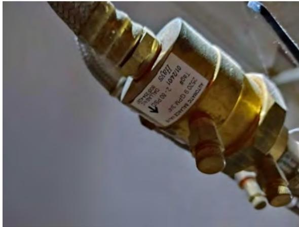
**Photo #121** Close-up view of auto balancing valve for WSHP.
