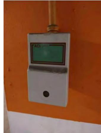
**Photo #160** Typical parking structure CO sensor for ventilation system.
