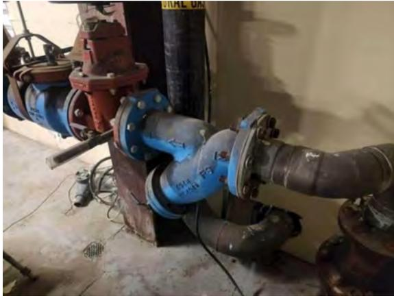
**Photo #105** Backflow preventer for main water distribution.
