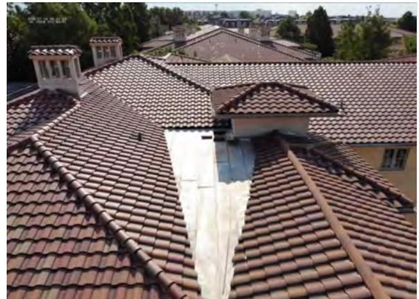
**Photo #28** View of standing seam metal roof in roof valley.
