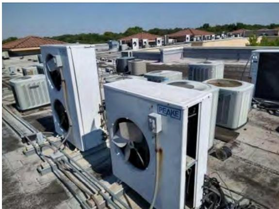
**Photo #113** Older DX split system condensing units on the roof.
