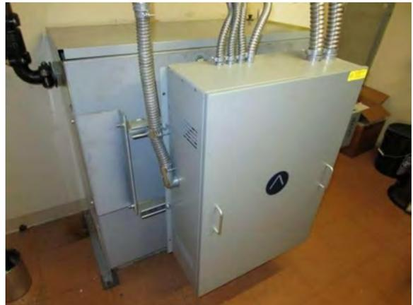
**Photo #136** Typical hydraulic elevator equipment.
