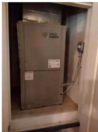
**Photo #119** Older WSHP (vertical orientation) in mechanical closet for dwelling unit.
