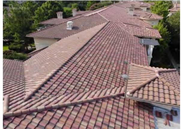
**Photo #20** Close view of concrete tile roof.
