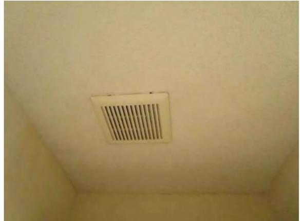
**Photo #130** Typical exhaust fan in dwelling bathroom.
