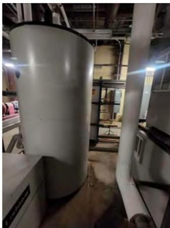
**Photo #101** Storage tank for domestic hot water.
