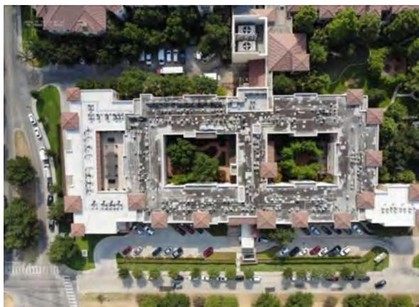
**Photo #29** Overview of modified bitumen roof over the entire Plaza building.
