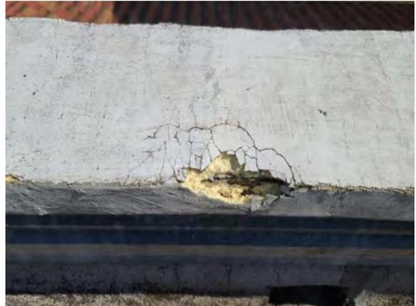
**Photo #52** View of damage to EIFS coping.
