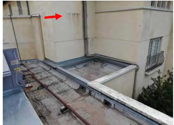
**Photo #50** View of staining on stucco façade.
