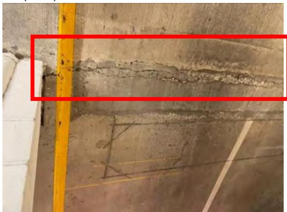
**Photo #59** Crack in deck along the joint between Phase II and Phase II in main parking structure.
