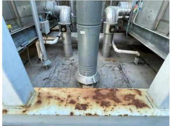
**Photo #62** Cooling tower structure shows deterioration.
