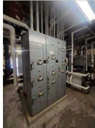
**Photo #104** Motor control center in central plant.
