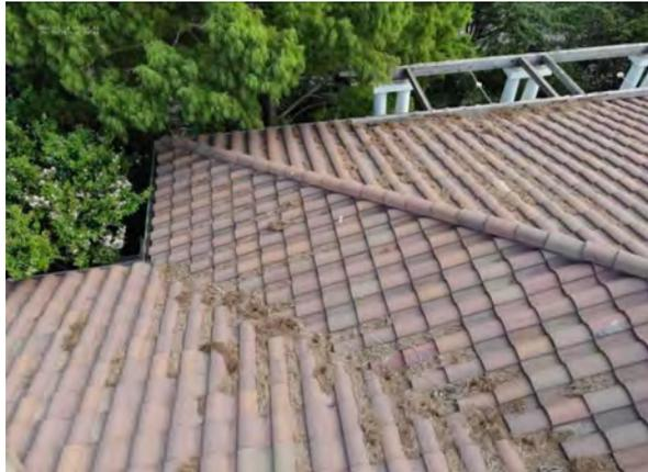
**Photo #25** View of debris build up on roof. Note tree encroachment of roof.
