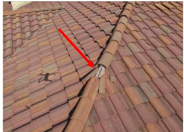
**Photo #24** View of broken tiles on roof. Located periodically through site.
